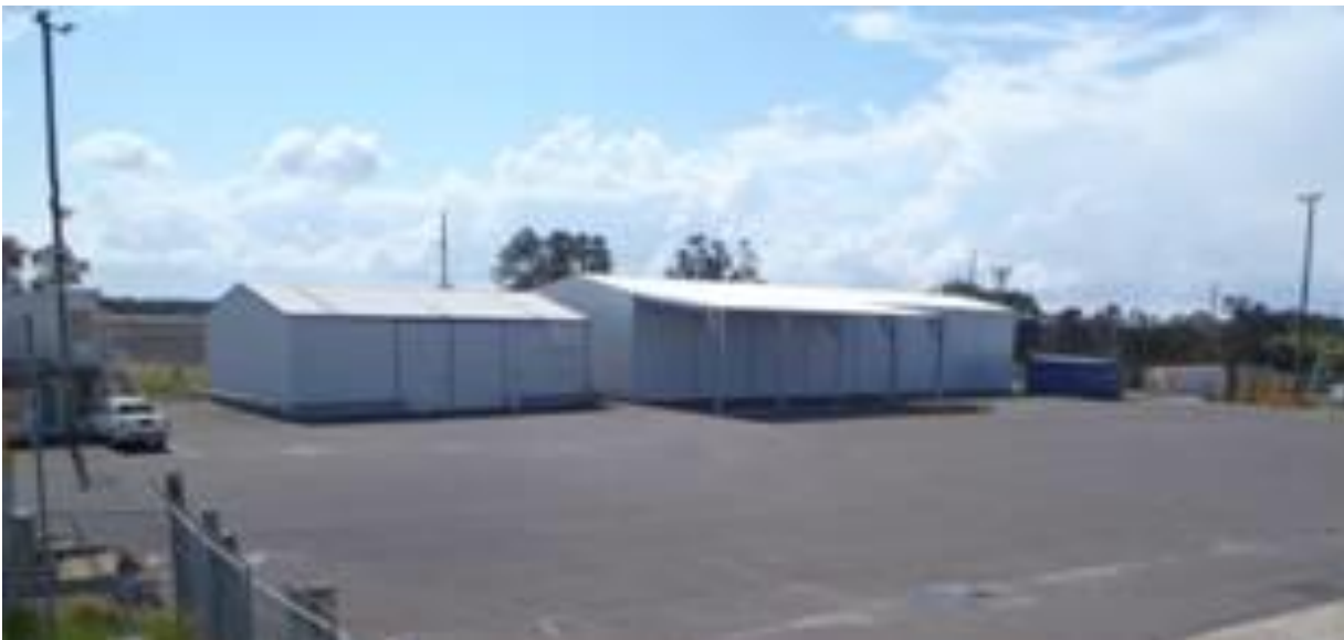
Goodwood Wharf – hard stand and lockable storage
