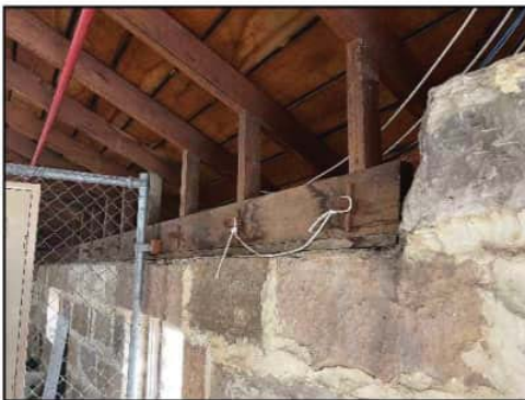
Figure 30. Internal view to the timber roof structure and framing.
