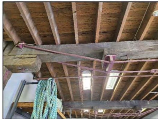
Figure 25. Internal view to significant timber beam.
