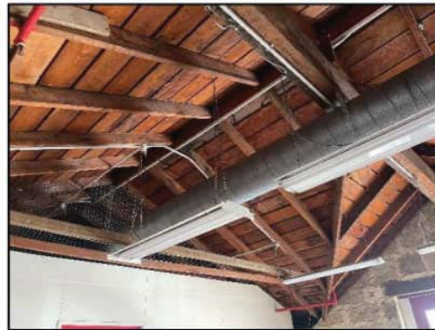
Figure 29. Internal view to the timber roof structure and framing.
