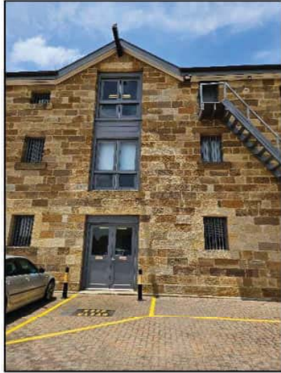
Figure 18. External view to details on the western elevation.
