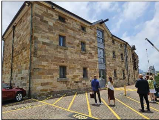
Figure 16. External view of the eastern elevation of the subject building, facing north-west.
