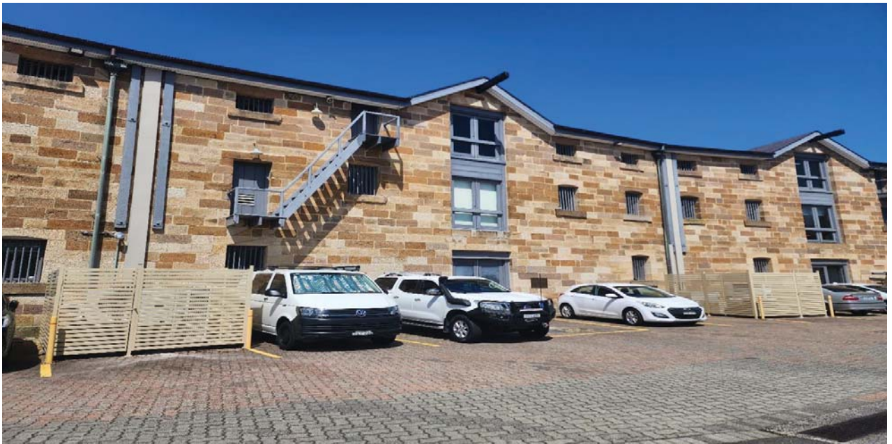
Figure 1-4 View of building west elevation, middle section is proposed area of the lift (Source: Worley, 2024)
