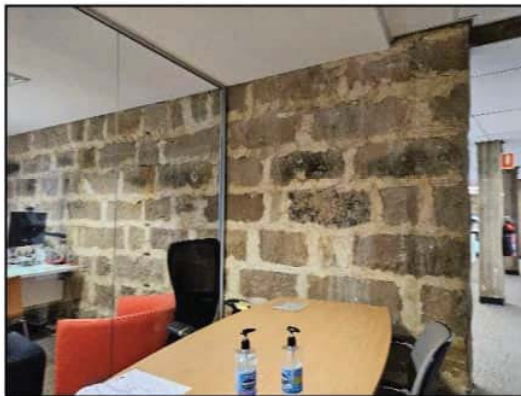
Figure 24. Internal view of original sandstone masonry.
