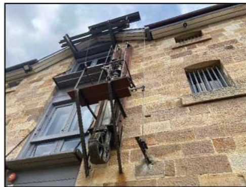
Figure 21. External view to the hoisting system on the eastern elevation.
