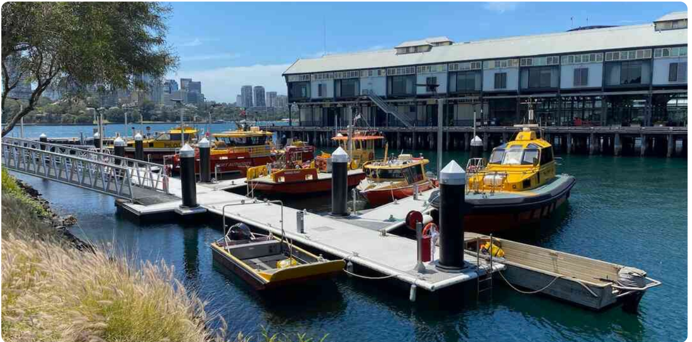
NEW FLOATING PONTOON AT MOORE'S WHARF
