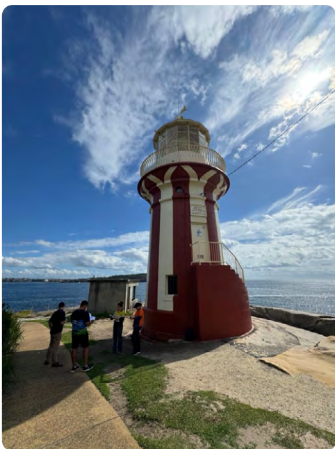
TECHNICAL INSPECTION CARRIED OUT AS PART OF THE PREPARATION OF THE ACHAR FOR THE PROPOSED WORKS AROUND THE HORNBY LIGHTHOUSE
