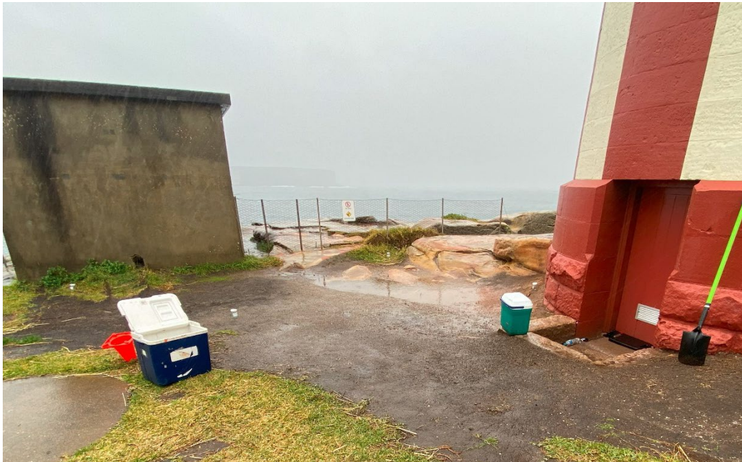
Plate 3 – View towards the north-east, showing the rocky outcrops on the northern side of the lighthouse.
