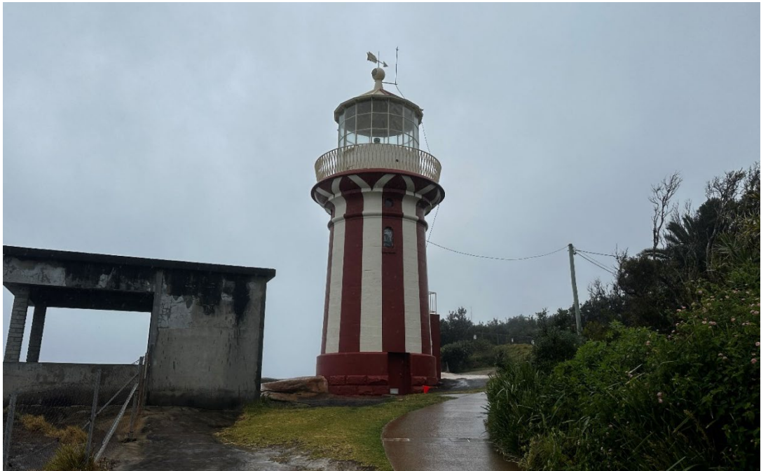
Plate 14 – View towards the south-east, showing the lighthouse, concrete structure, garden beds and the pavement.
