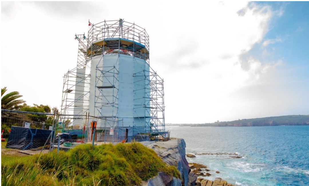
Plate 8 – Photograph dated 2024 (Source: Facebook Page of Bayside Scaffolding Services).
