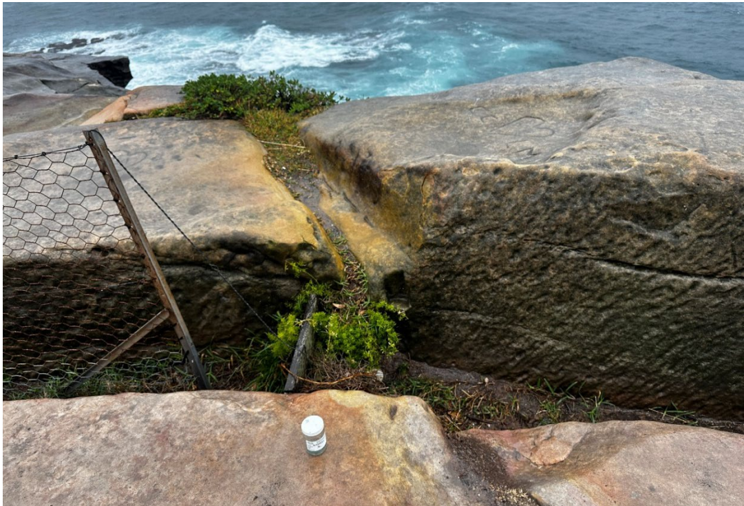
Plate 16 – View of the sandstone wall surrounding the lighthouse, showing the soils within the crevices.
