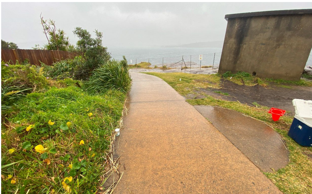
Plate 13 – View towards the north along South Head Heritage Trail, showing the concrete structure and garden beds to the west.
