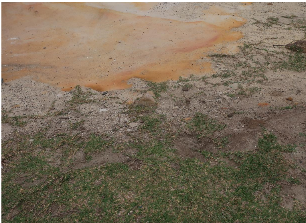
Figure 6-2 View of ground exposure. Located west of Lighthouse, looking north. AMAC Group, 11/11/2024, Image No. 091026.
