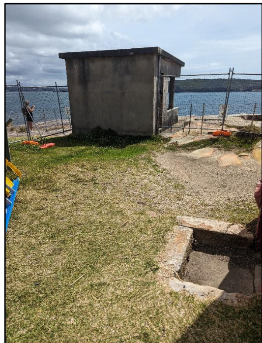
Figure 7. External view to the area of works, facing north.
