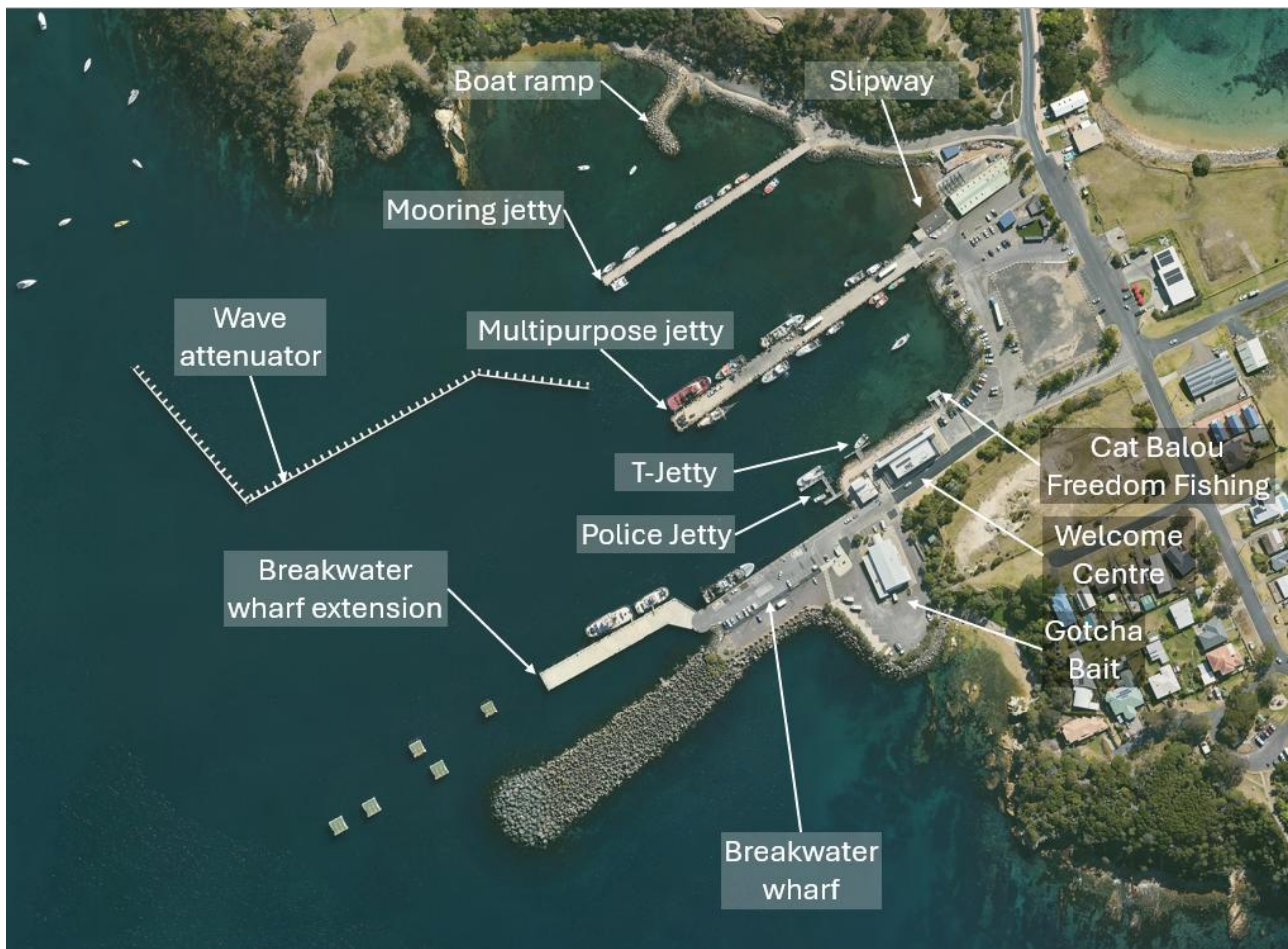
Figure 3: Eden Cruise Wharf(or Breakwater Wharf Extension) within its context in Snug Cove, Eden (Source: MetroMap, Sep 2023)
