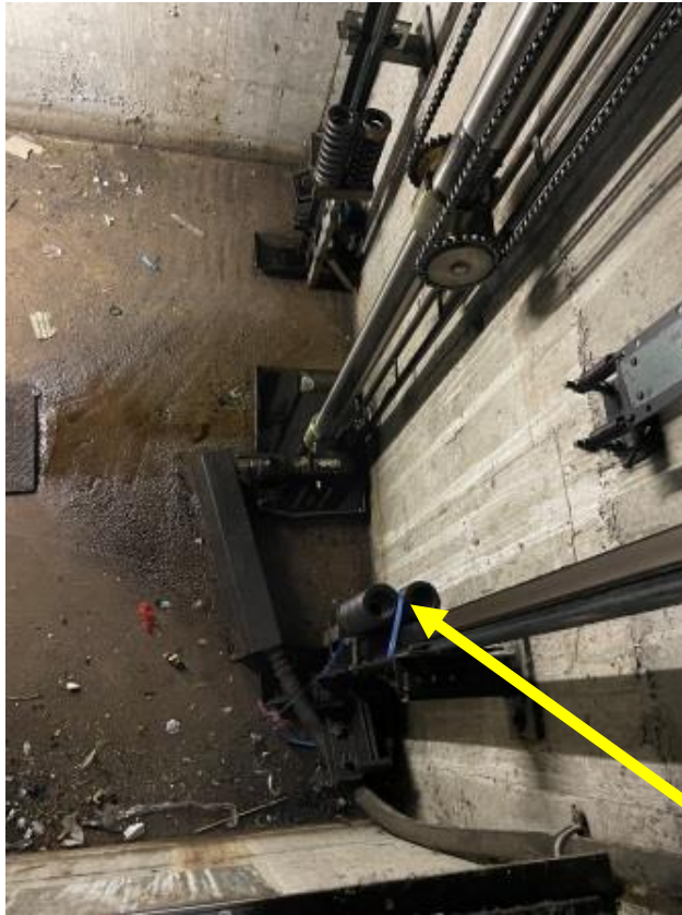
Lift 5 – excess oil needs to be cleaned from the lift pit floor and the floor degreased. The hydraulic ram needs new seals.
