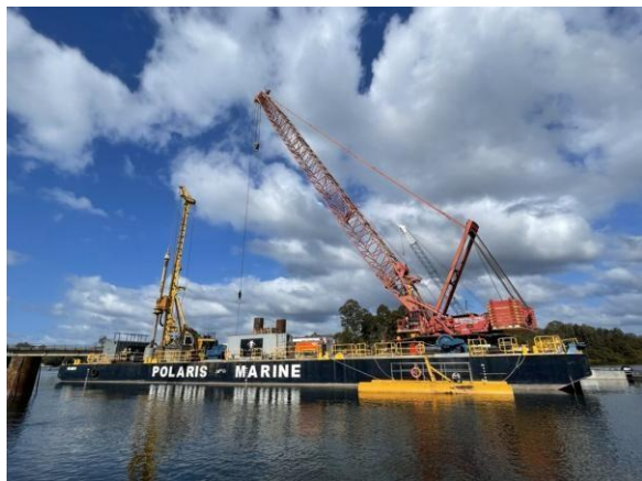
Figure 4: 53m PM East Crane Barge
