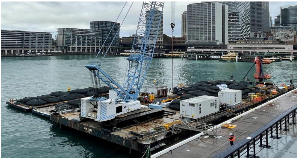
Figure 2: Crane barge with scour protection bags
